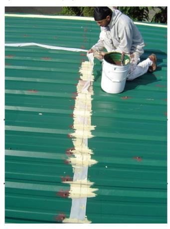
Reinforcing mesh is applied to all remaining standing seams. A second, thick coat is applied to the surface to fully embed the mesh and eliminate all pinholes. Since RD products are thixotropic, they can be applied in thick coats without slumping.
