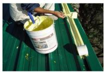
Once all the seams and exposed screws have been detailed with RD-Elastometal, the body of the metal roof is ready to receive the spay application of RD-Elastometal.
