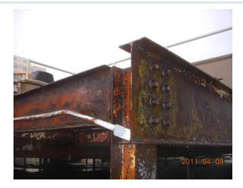
Above photo is after surface preparation of 5,000psi Using the zero degree turbo tip.
