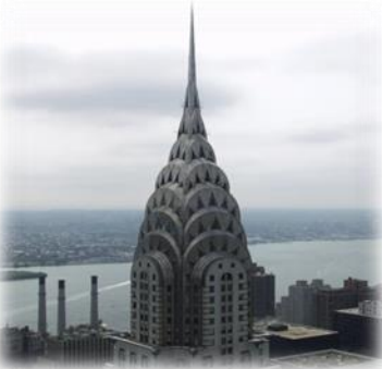
The Chrysler Building in New York City made use of RD-Elastometal and RD-Mur Acryl to renovate and repair the stainless steel spire.
