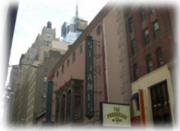
The St. James Theatre in New York City used RD-Elastoflex to complete its Restoration
