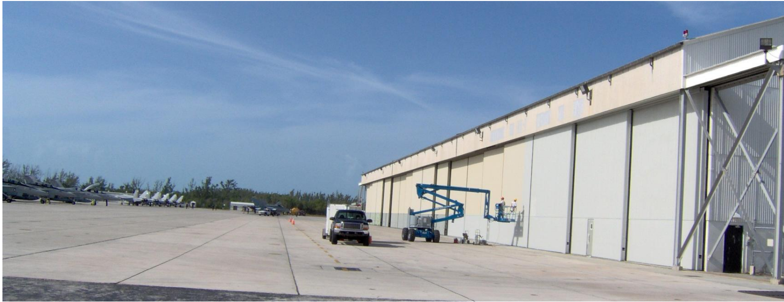
APPLICATION OF SECOND COAT RD-ELASTOMETAL.
