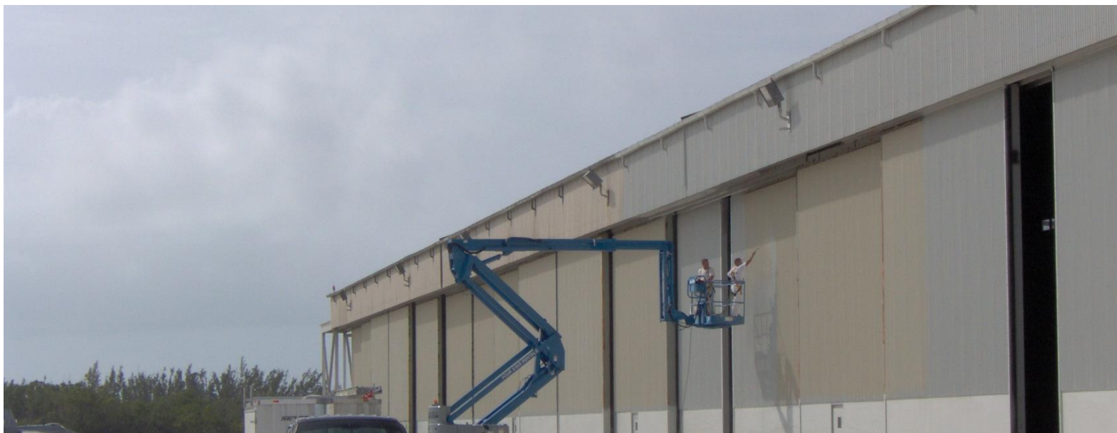
APPLICATION OF FINISH COAT RD-MUR ACRYL.
